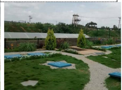
Overview of plant
