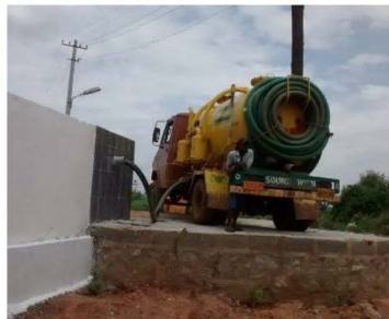
Fecal sludge being discharged
